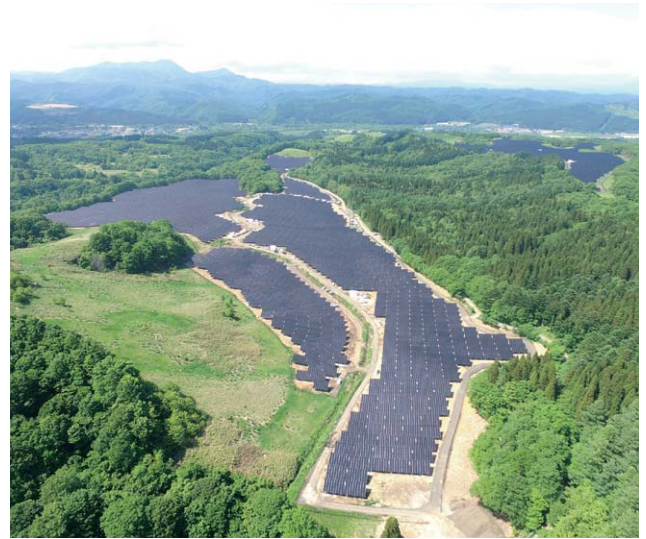
Hokkaido SHIRIUCHI MEGA SOLAR 20M Power Plant
