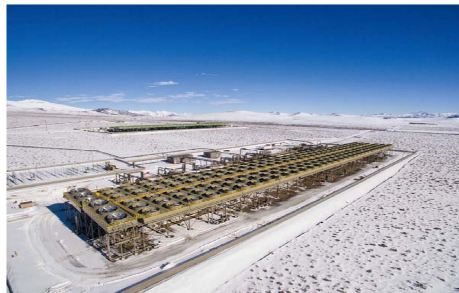
McGinness Hills Complex発電所
