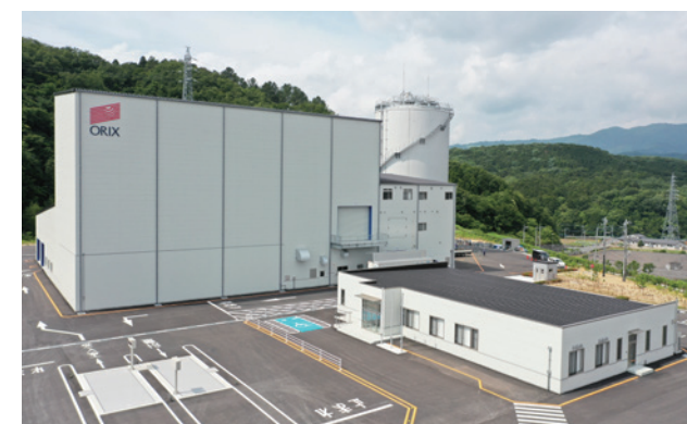
Biogas Power Generation Facility (ORIX Environmental Resources Management, Yorii Biogas Plant)
