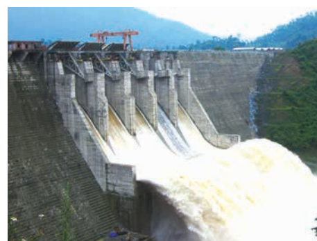
The Dak Mi 4 Power Station which is owned and operated by BPC
