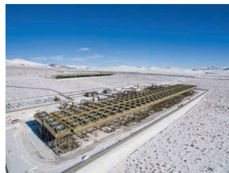
The McGinness Hills Complex Power Plant owned and operated by Ormat
