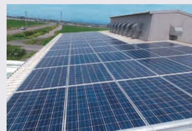
Saga Prefecture Fishery Cooperative Federation, Hayatsue Branch Office, Cooperative Facility (Saga, Saga Prefecture)
