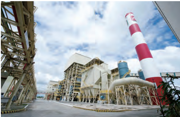
Power Plant on Panay Island
