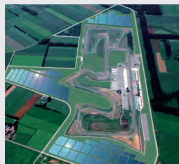
Image of completed project
