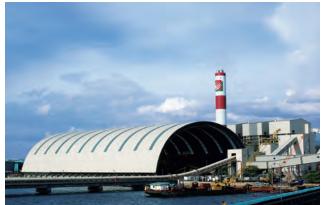
Power Plant on Cebu Island
