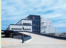
The Iwatsuki Logistics Center (Awarded CASBEE Saitama Prefecture Class A Rating)
