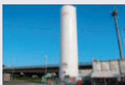
LNG satellite tank introduced at the Hokkaido plant
