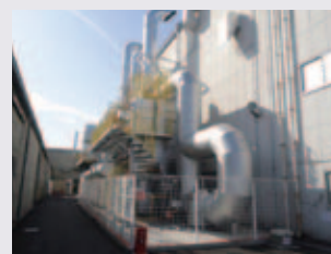
VOC processing equipment (RTO) installed at the Tokyo plant of the Ueda plant
