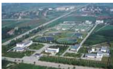
Sewage treatment facilities managed by China Water Affairs Group (Jingzhou City, Hubei Province)
