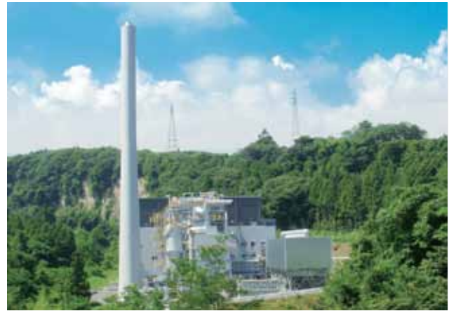
Agatsuma Biomass Power Plant
