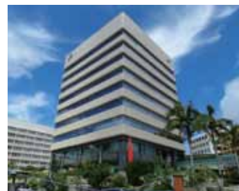
Okiden Naha Building
