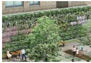
Artist's rendition of Sanctus Yono's greenery-covered walls (achieved CASBEE Saitama A-rank certification)
