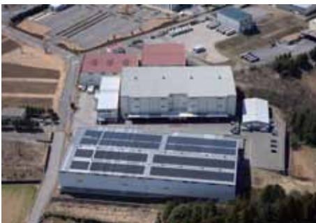
Roof of Fuji Logicargo's warehouse equipped with 2,300 solar panels (maximum output of 345.8kW)
