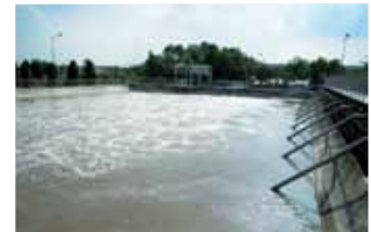
Sewage treatment facility
