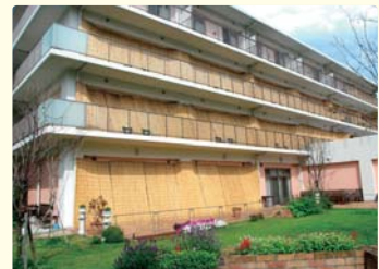
Reed blinds shading windows at Good Time Living Shin-Urayasu
