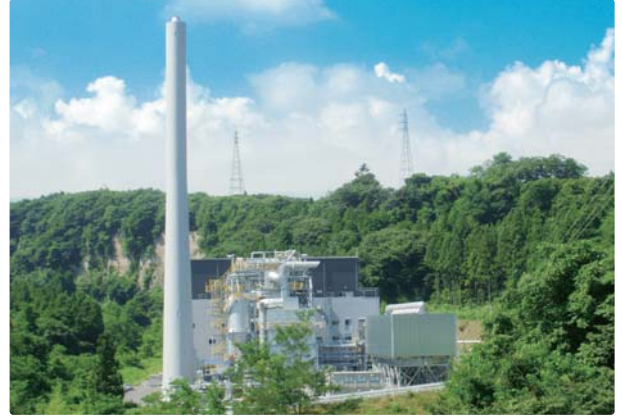
Agatsuma Biomass Power Plant
