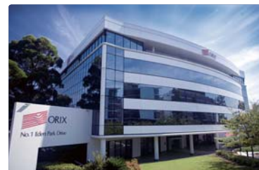
OACL's headquarters building, where electric power-saving measures are being implemented.
