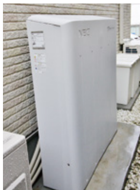
Installed storage battery
