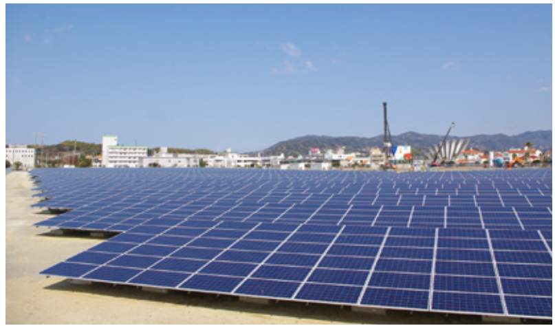
ORIX Awaji Mega-Solar Power Plant (Awaji, Hyogo Prefecture)
