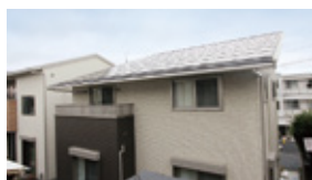
Rooftop solar panels
