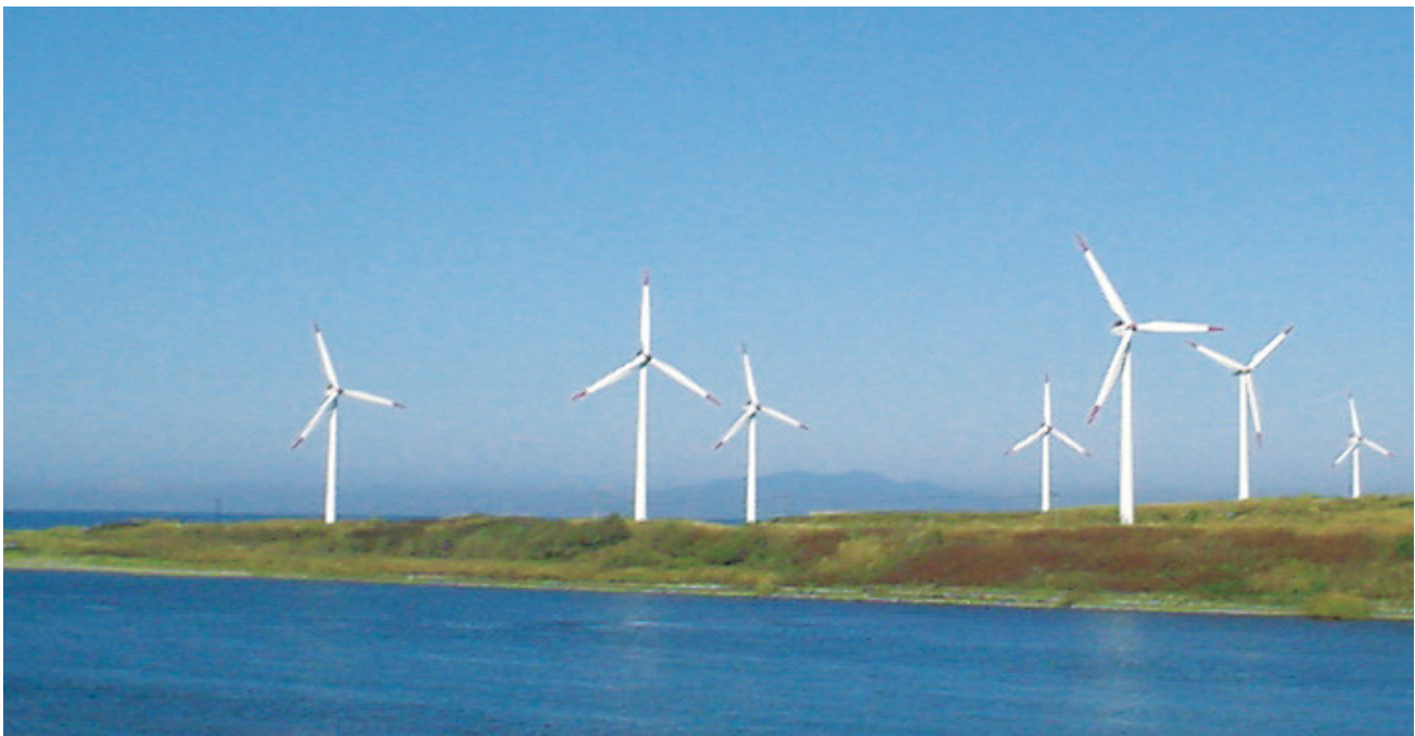
Akita Araya Wind Farm
