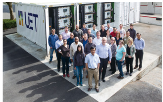
A large-scale energy storage system and local employees
