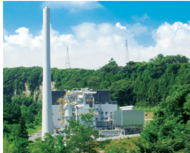
Agatsuma Biomass Power Plant
