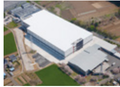
Moriya Logistics Center
