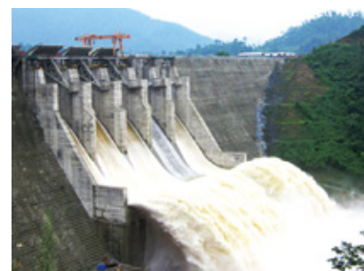
The DakMi 4 power station which is owned and operated by Bitexco Power Corporation
