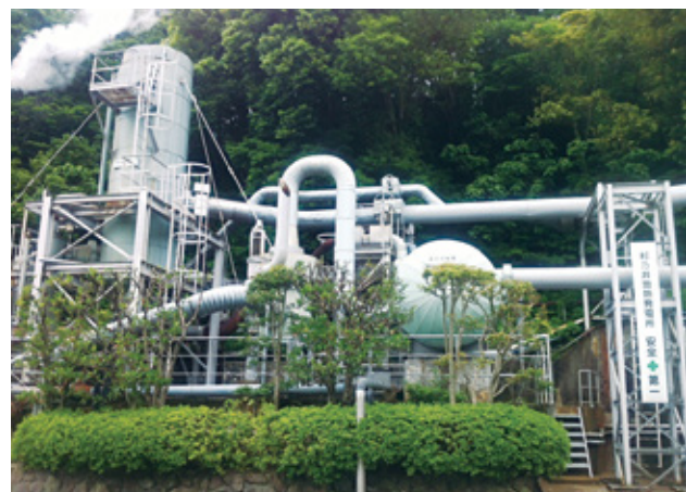
Suginoi geothermal power generation facility
