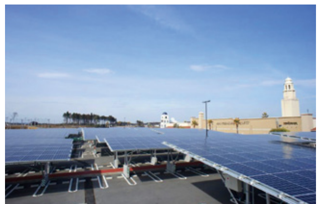
Carport-type solar power generation systems
