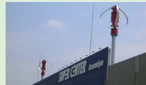
Wind power generation
