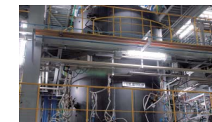
This high-temperature reactor furnace is the heart of the facility's waste decomposition system. Gas recovered from waste processed at temperatures of up to 2,000°C is reformed and used as a fuel for power generation.
