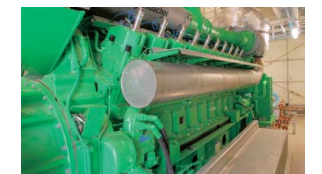
This gas engine achieves highly efficient power generation, creating up to 8,000kW of surplus power through the operation of parallel gas turbines.
