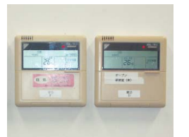
Remote controls for air conditioning units
