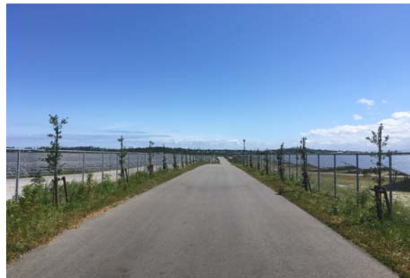
Improvement of nearby roads
