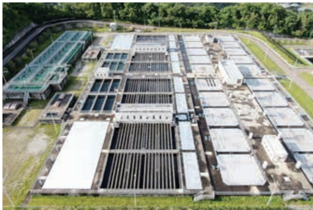
Nanbuyama Water Treatment Plant (Shiroishi City, Miyagi Prefecture)
