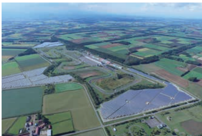
ORIX Sarabetsu-Tokachi Mega-Solar Speedway Power Plant
