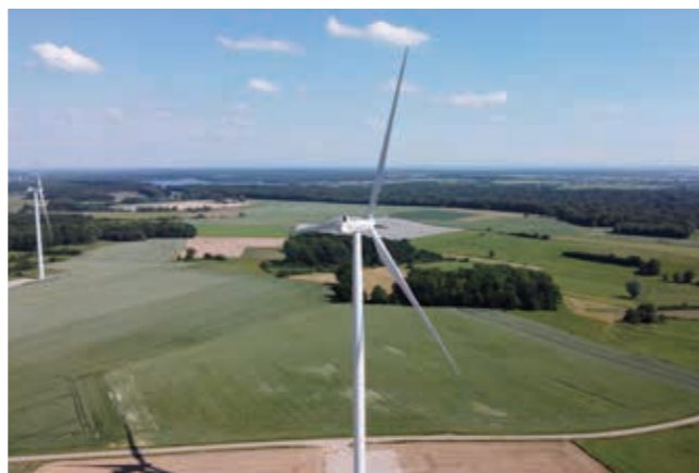
Wind power generation facility operated by Elawan Energy
