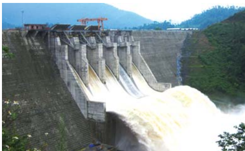
The DakMi 4 power station, which is owned and operated by BPC
