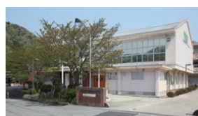
Plant factory using a former gymnasium of an elementary school
