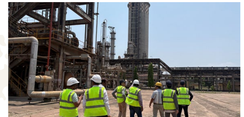
Proposed site for a green ammonia production facility
