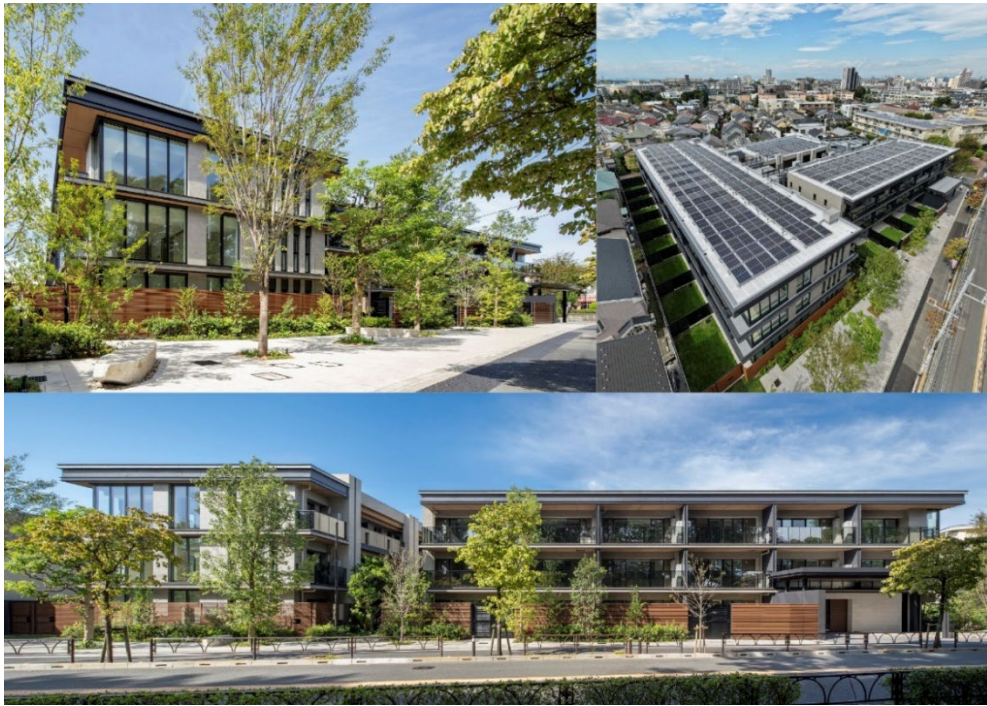
Exterior of “The Lions Setagaya Hachimanyama” and Its Rooftop Solar Power Generation Equipment
