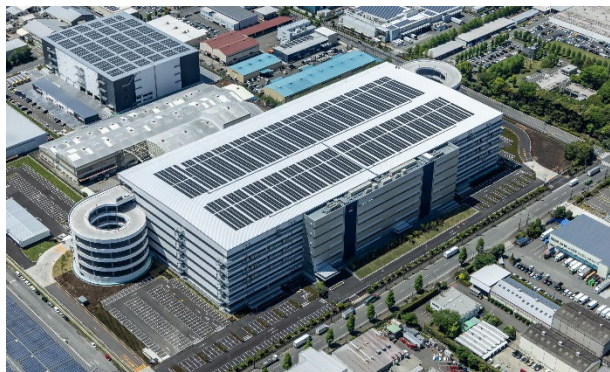
Exterior of the facility (aerial photo)
