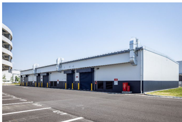
Dangerous goods warehouse
