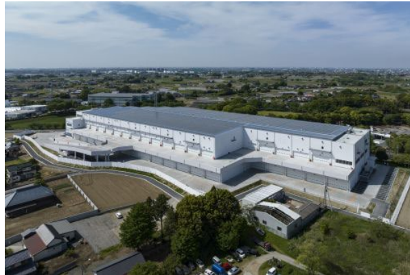
Exterior of Kazo Logistics Center
