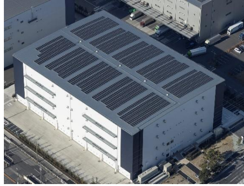
Solar power generation system installed on the roof
