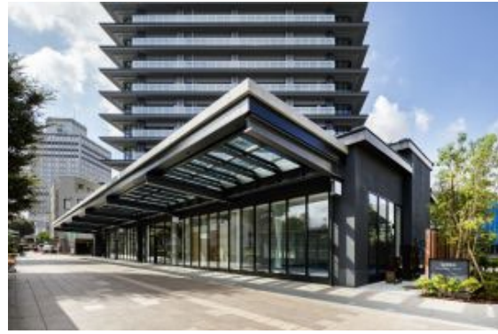
Eaves of the arcade
