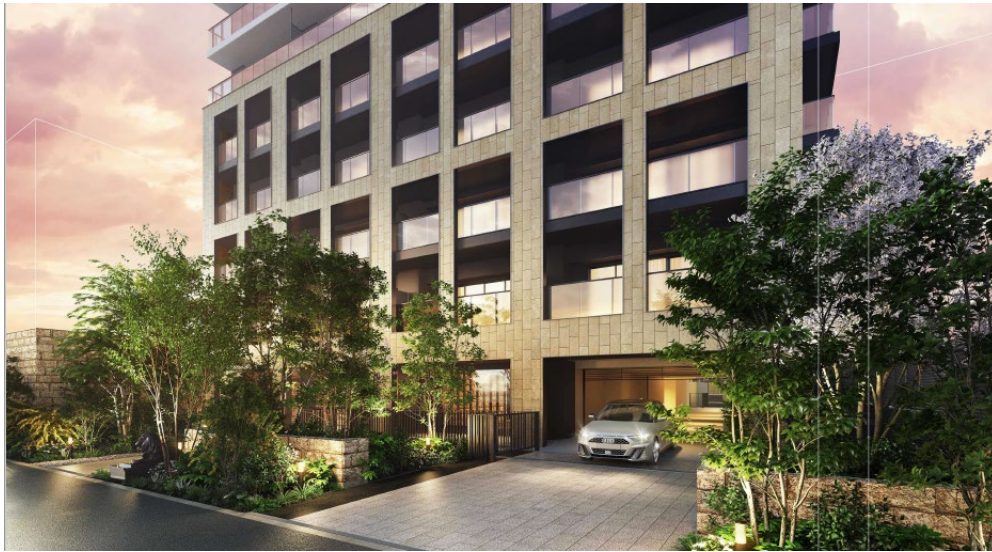
Image of the exterior
