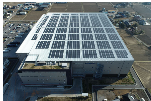
Installed solar power generation system
