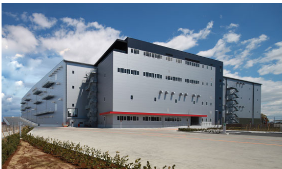
Exterior view of Matsubushi LC
