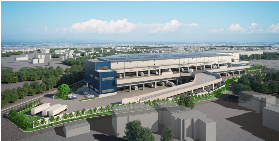
Exterior image of Kazo Logistics Center
