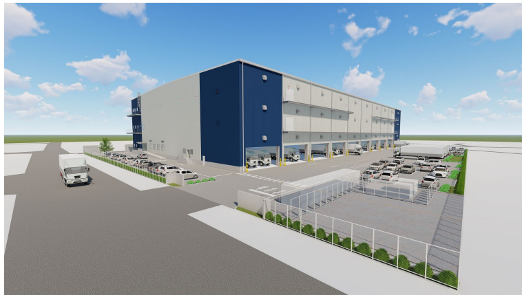
Exterior image of Moriya II Logistics Center
