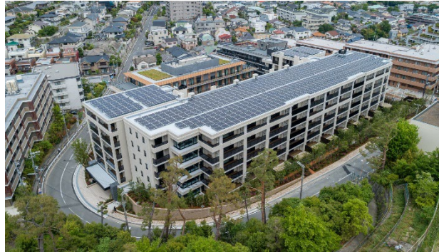
Building exterior and rooftop solar panels
