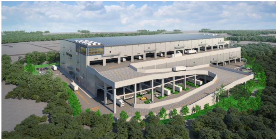
Exterior image of Tsurugashima II Logistics Center
