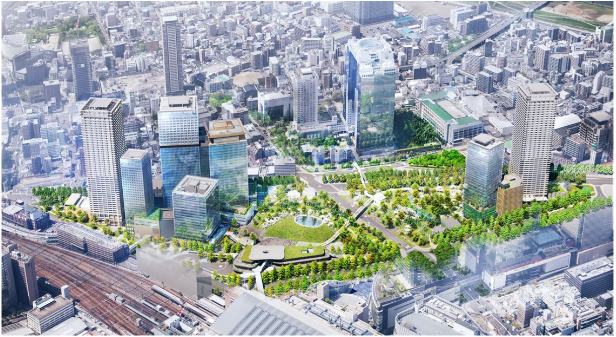
Panoramic view of Umekita 2nd Zone (Concept image for completed project) * Subject to change
