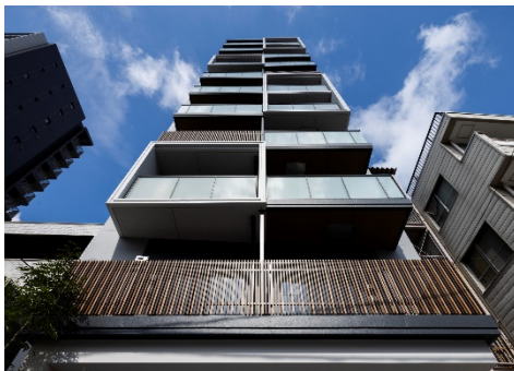
Building exterior of Lions Forsia Takanawa
