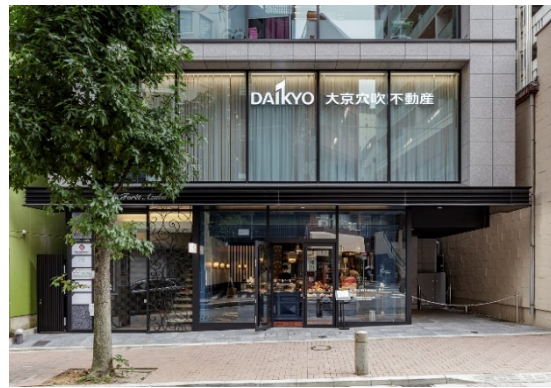
External appearance (2 nd floor)
