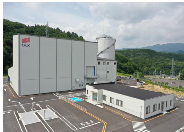
Yorii Biogas Plant
