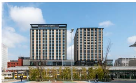
The exterior of CROSS GATE KANAZAWA
