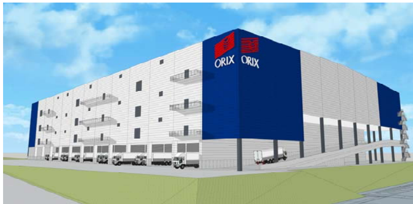
Exterior of the Minoh Logistics Center (tentative name)
