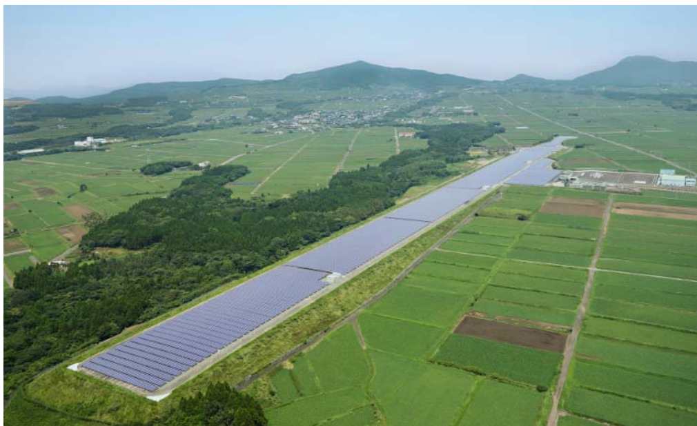
Makurazaki Former Airport Site No.1 and No.2 Power Plants
