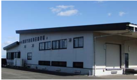
Seaweed Collection Facility (Kashimashi, Saga Prefecture)
