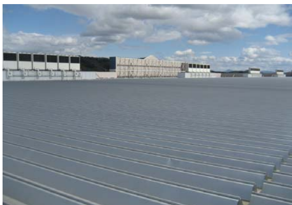
PLANT-5 Otama Store (Rooftop)
