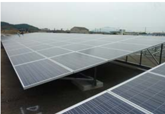
Solar Panel Installation Fukushima Prefecture
