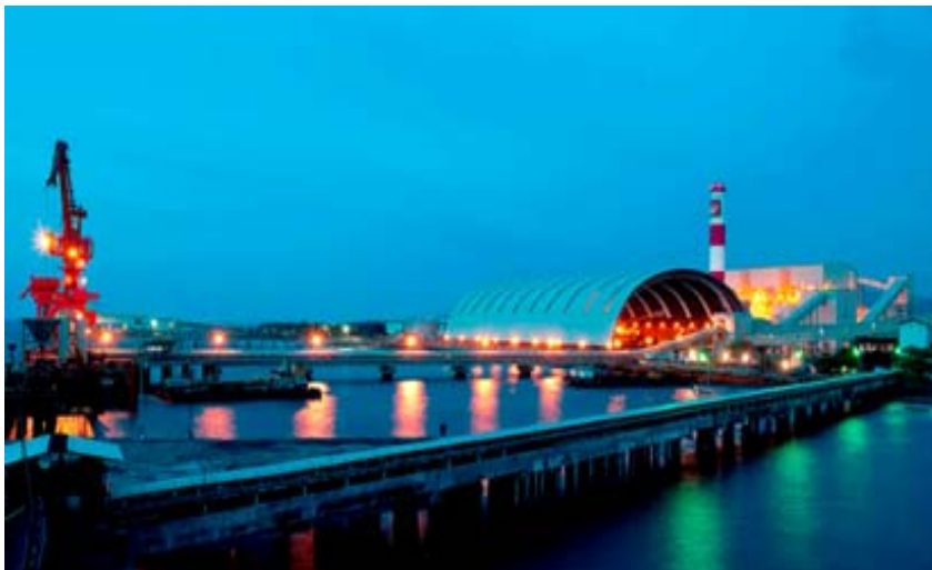
Power Plant (Cebu Island)
