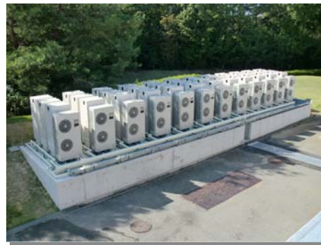
Multi-split outdoor air conditioning system for building use (left) and heat pump water heating equipment (right) at Fuji OGM Golf Club Ono Course
