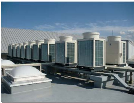
Multi-split outdoor air conditioning system for building use (left) and heat pump water heating equipment (right) at Fuji OGM Golf Club Ono Course
