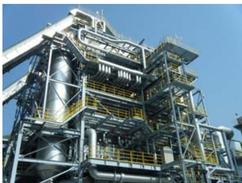
Internally circulating fluidized bed boiler
