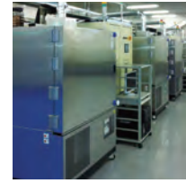
Charging and discharging testing equipment
