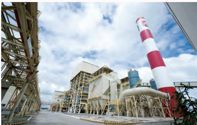
Power Plant on Panay Island
