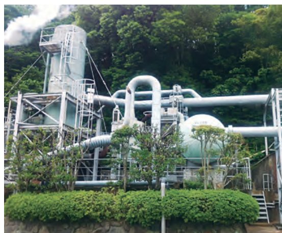
Suginoi geothermal power generation facility
