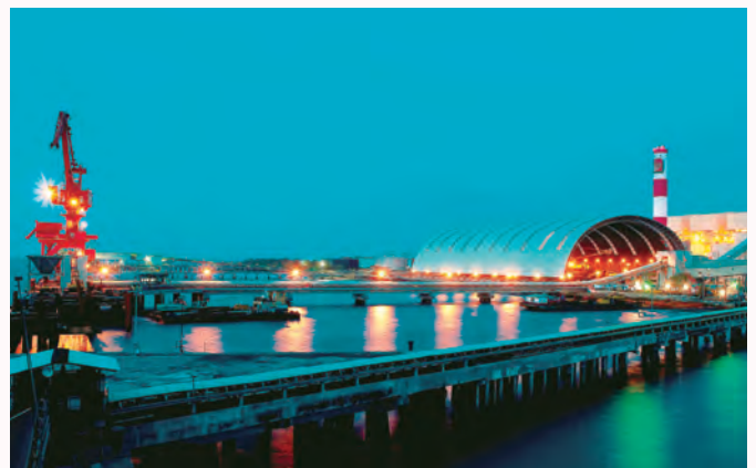
Power Plant on Cebu Island
