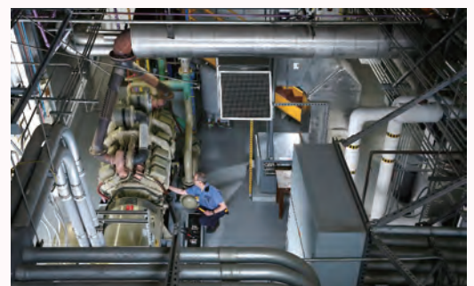
Maintenance work on power generation facilities installed in an office building basement
