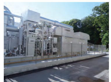
Co-generation system installed at the Takasaki Plant
