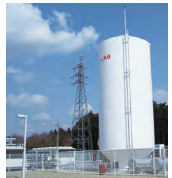
LNG satellite tank introduced at Mochida Pharmaceutical Plant's head office plant
