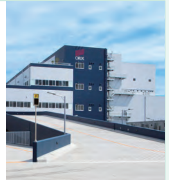
The Iwatsuki Logistics Center (Awarded CASBEE Saitama Prefecture Class A Rating)
