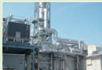
Gas turbine power generator at Otsuka Chemical's Tokushima Plant
