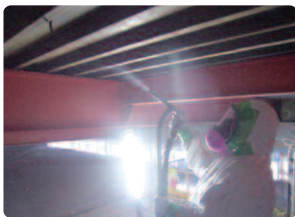
Dry ice blast
