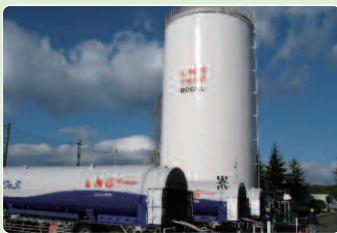
LNG satellite tank installed at Sumitomo Rubber Industries' Shirakawa Factory
