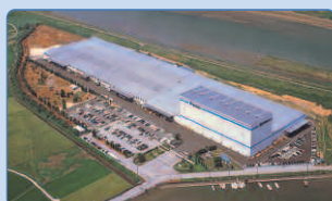
Daiwa Industries' Saiki Plant
