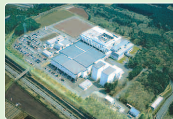
The Head Office Plant of Mochida Pharmaceutical Plant Co., Ltd. is switching to LNG fuel.
