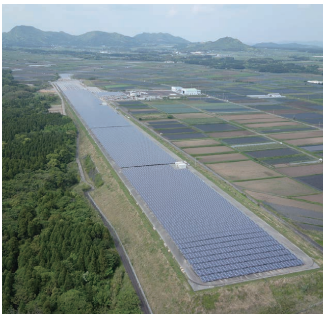
Mega-solar power plant built on the former site of Makurazaki Airport in Kagoshima Prefecture
